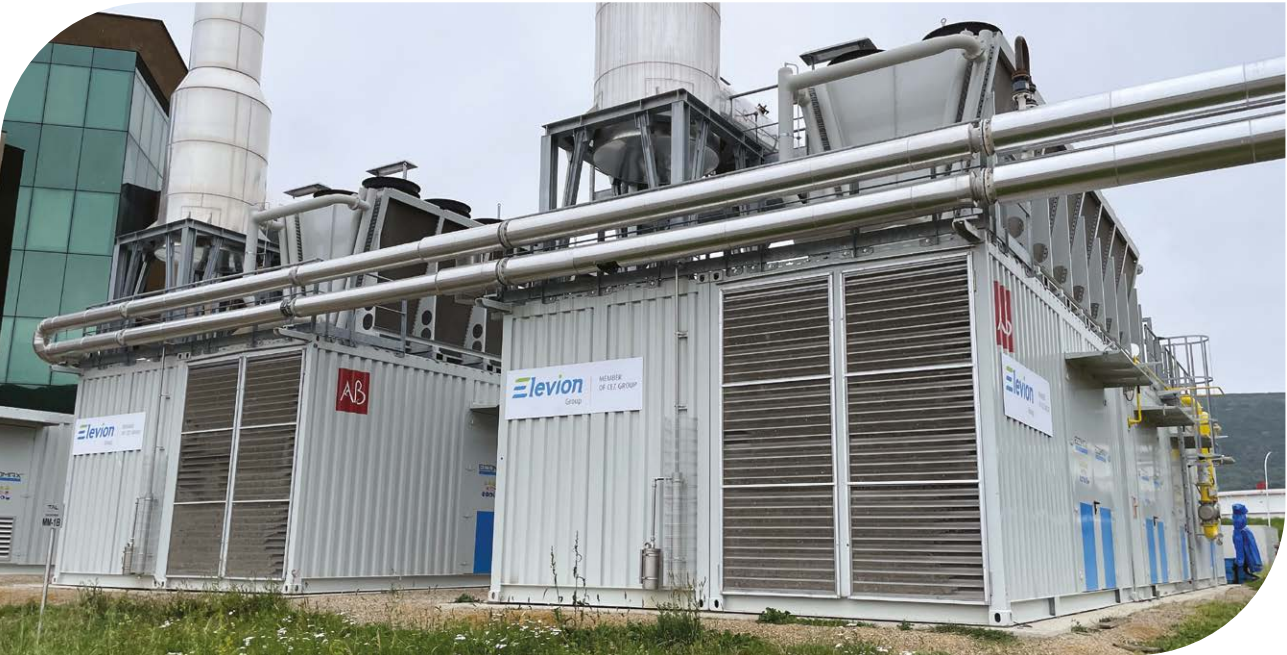
High efficiency cogeneration units along the TAL pipeline, Italy, Elevion Group
